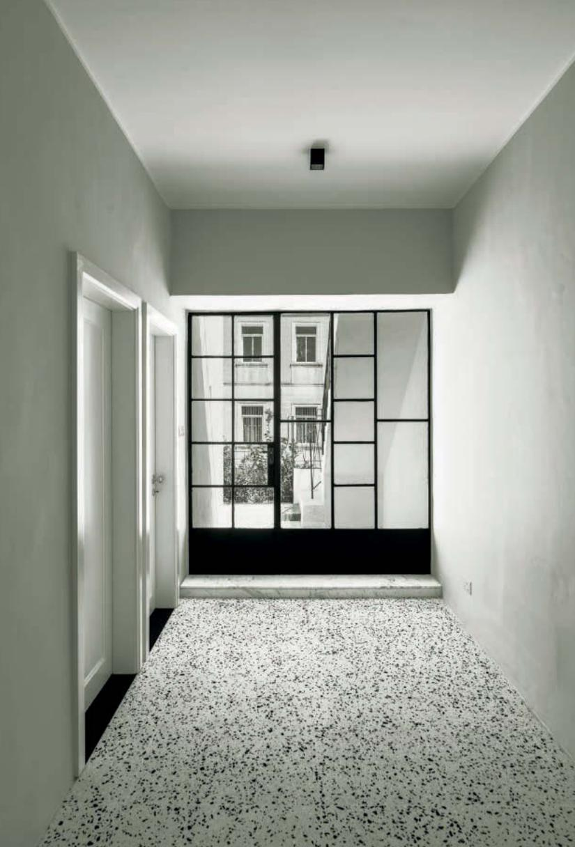
Since the flooring varied from one room to the next, a monolithic, solid black, quartz sill was installed to serve as a threshold beneath each internal door, further emphasising the length and width of the corridors.
